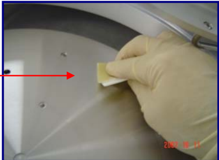
Fig 11 & 12: Lightly dampened ScrubPAD scrubbing top of Degas Heater
