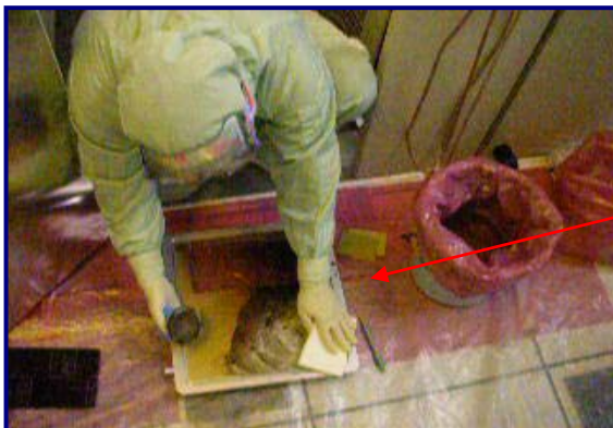
Fig 8 & 9: Lightly dampened UltraSOLV ® Sponge wiping away excess deposition
