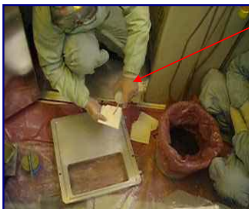
Fig 26: Saturating HT5790S MiraWIPES® with IPA
