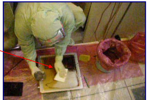
Fig 8 & 9: Lightly dampened UltraSOLV ® Sponge wiping away excess deposition
