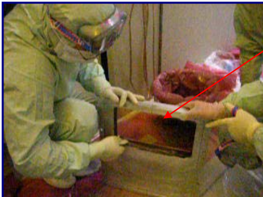
Fig 19: UltraSOLV® Sponge removing excess deposition from lip of chamber door
