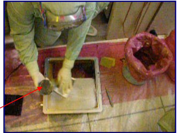
Fig 14: Wiping away excess deposition with UltraSOLV ® Sponge
